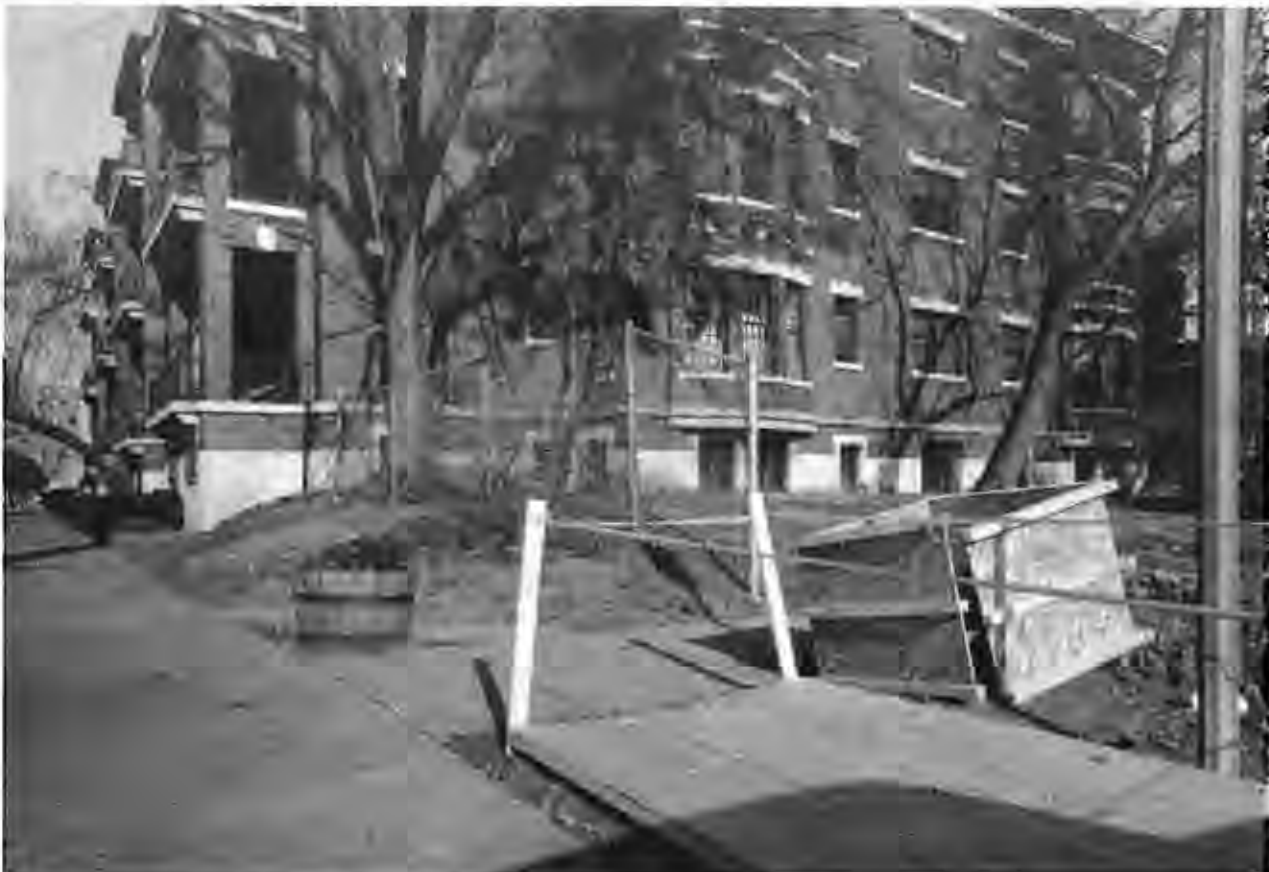
Work begins on foundations for entrance pillars along Skinker, here at Pershing.
